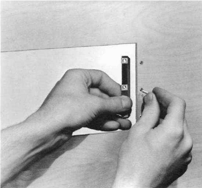
Insert the screws in the center holes of the cabinet panel ("B" holes on the template) and tighten. The screw head should pull into the wood slightly. (Use two  $\frac{3}{4}$  inch long screws for panels under  $\frac{1}{2}$  inch, or two  $1\frac{1}{4}$  inch long screws for panels  $\frac{1}{2}$  inch thick and larger.)
